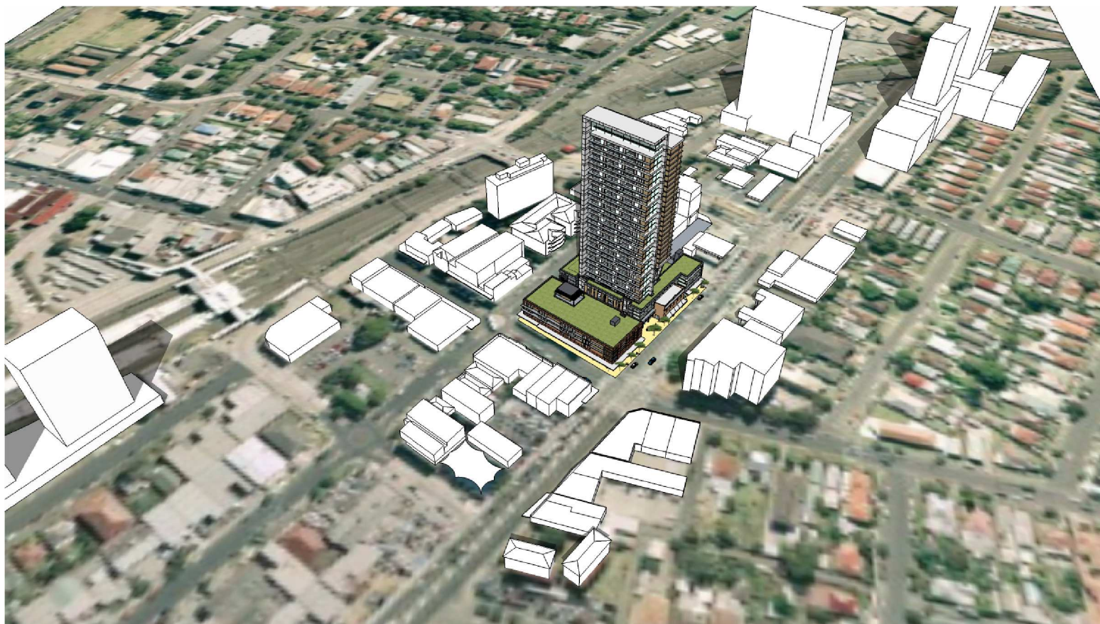
NORTH-EAST AERIAL VIEW
